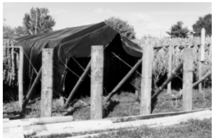
Figure 3: End-post bracing and plastic covering for high-tensile structure.
