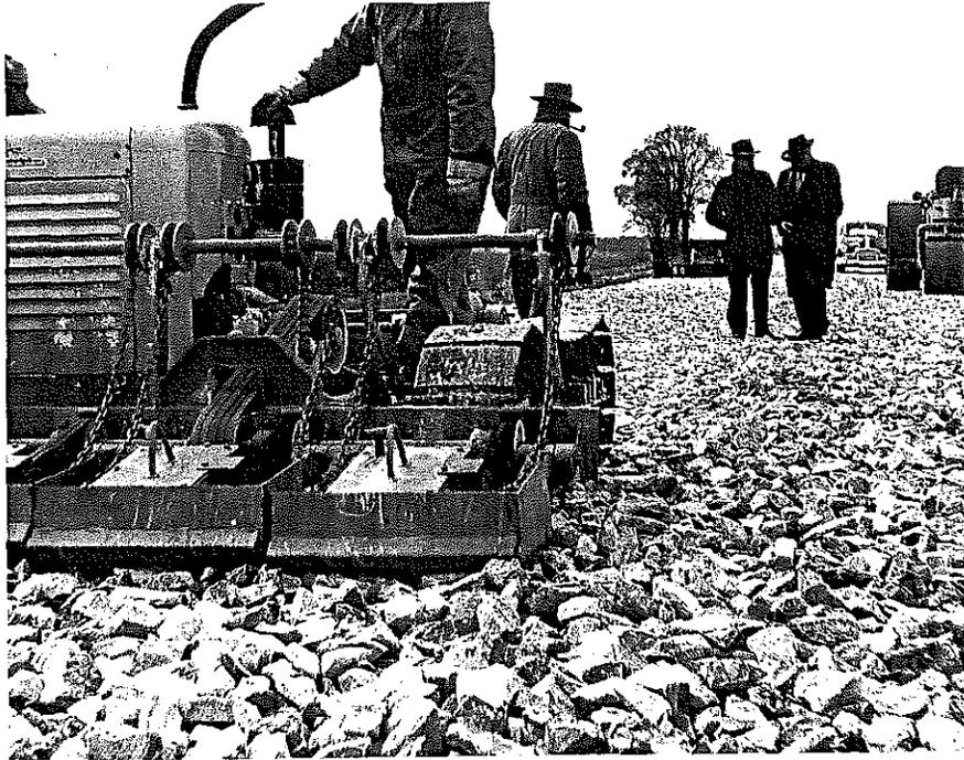
Fig. 3. Initial compaction of the loose stone was obtained with the vibratory tamper rather than the three-wheel roller. Here the tamper is shown compacting loose stone, the effect of which is shown by the contrast between compacted material behind the machine and loose material on the right.
