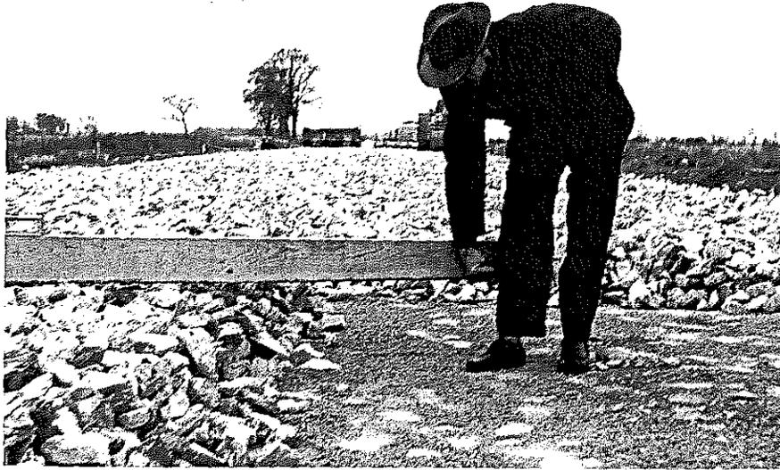
Fig. 2. Coarse stone for the base contained an unusually high percentage of elongated pieces, as can be seen at several points in this photograph. This was not particularly detrimental in the spreading or compaction of the material, and the base was well keyed when final compaction was completed. Note the indicated depth of loose spread.
