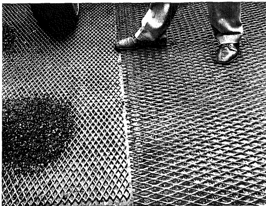
Fig. 3. Near view of abutting mats showing the 6 x 8 foot size on the right with mesh running transversely, and the 4 x 8 foot size on the left with mesh running longitudinally. Some of the smaller sheets were placed with the mesh running transversely (see Fig. 2). This view is toward the paver and away from the intersection.
