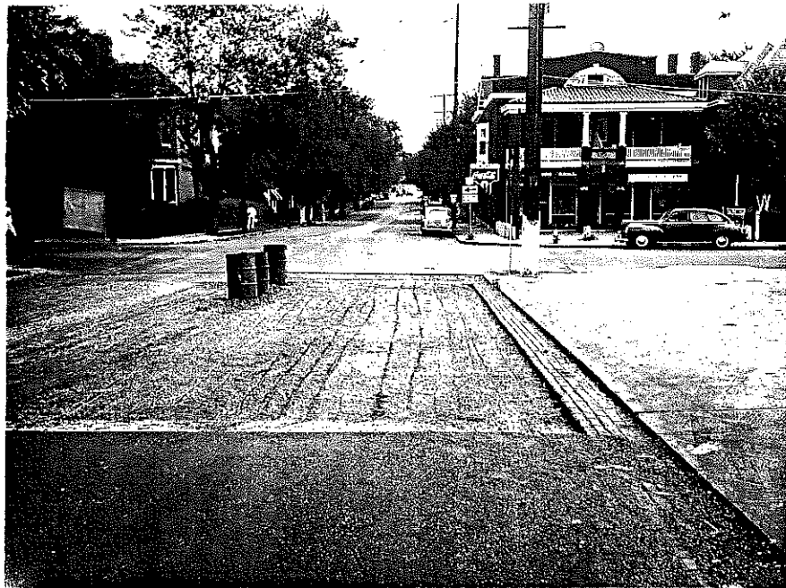
Fig. 1. Looking north on Jefferson Street into the intersection with Third Street. Here the old sheet asphalt pavement has been removed down to the original brick in preparation for the new pavement and the metal mats.
