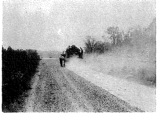
Fig. 8 - Champion Spreader in Operation, Excessive Application .
