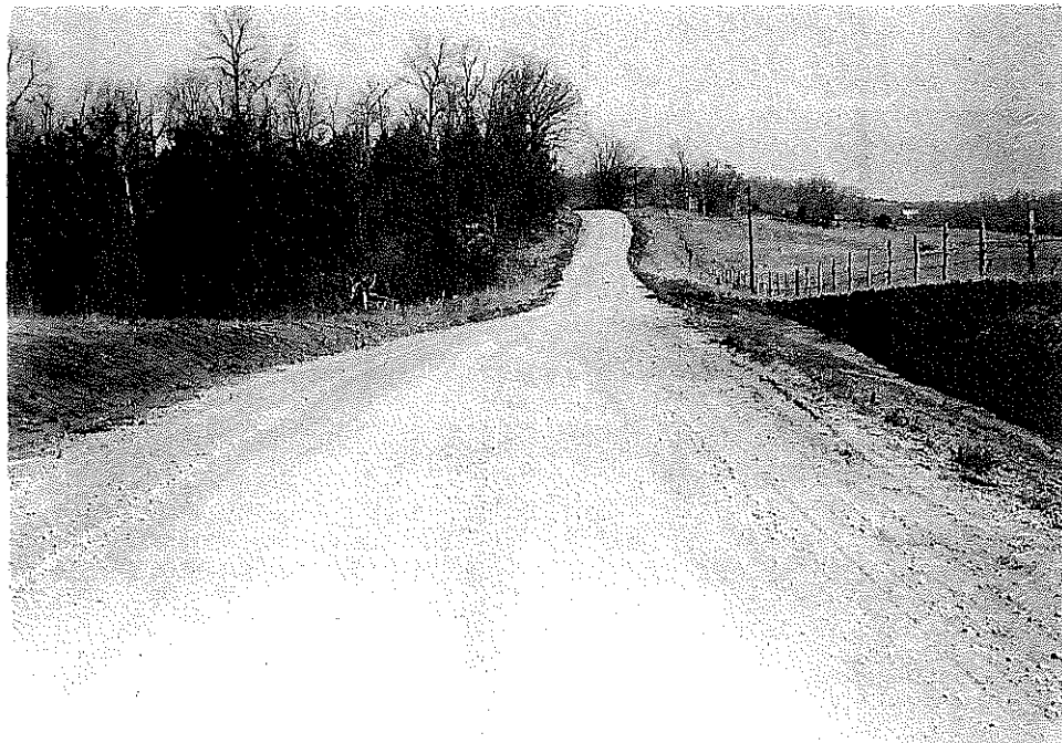
Fig. 14 - M.P. 100-25-C, Result of Sufficient Binder and High Crown, April, 1959.
