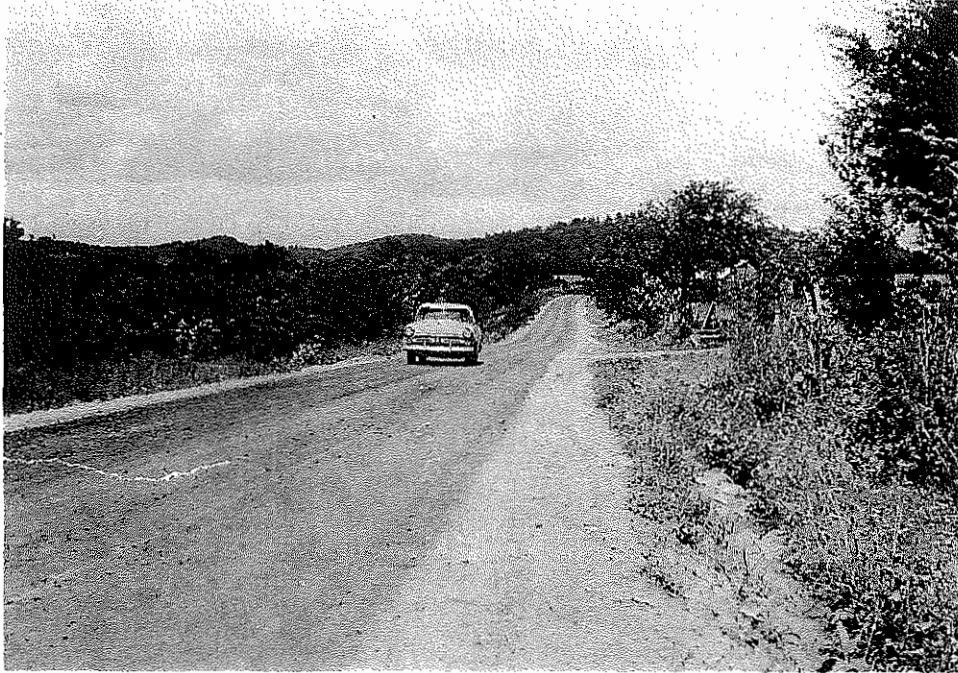
Fig. 15 - M.P. 100-855-E, Absence of Crown, August, 1958.
