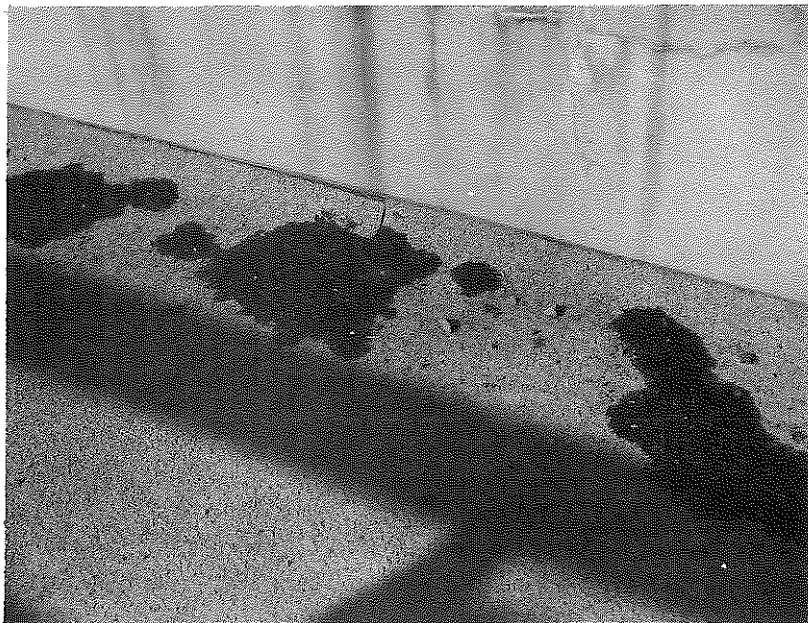
Figure 6. Close-up Showing Joint at Fillet of Curb. Note Slight Unevenness of Installation.
