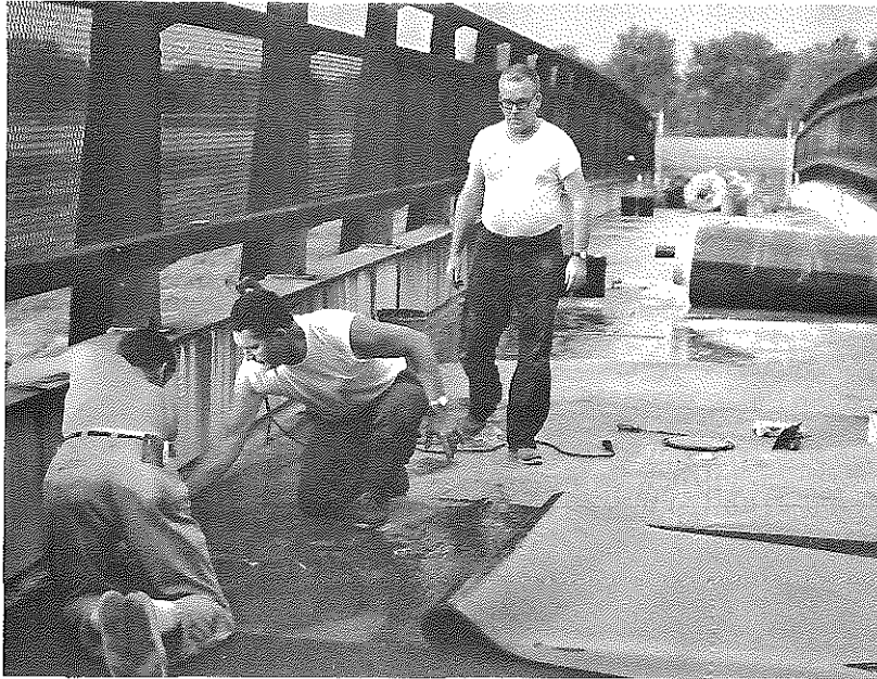
Figure 3. Laying Tartan Surfacing on the Bridge Deck.
