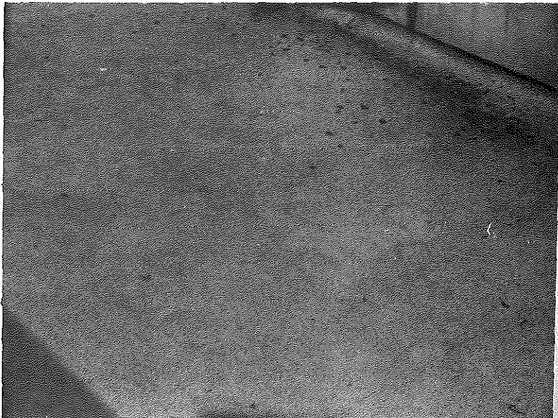
Figure 8. Horseshoe Tracks on Tartan Surface (4-25-73).
