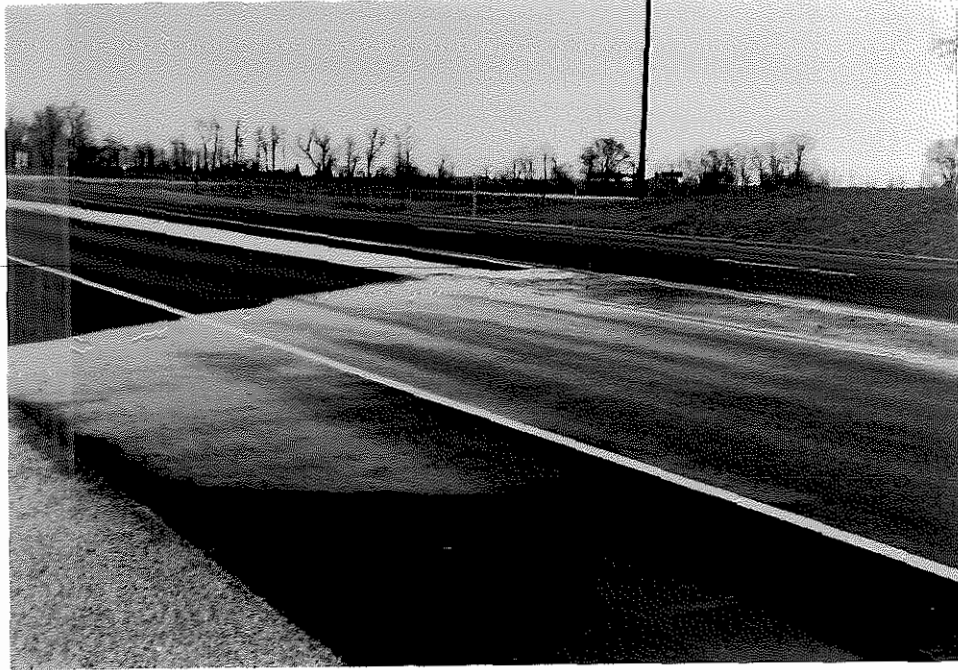
Figure 5. View Showing Superelevation, Southern End.
