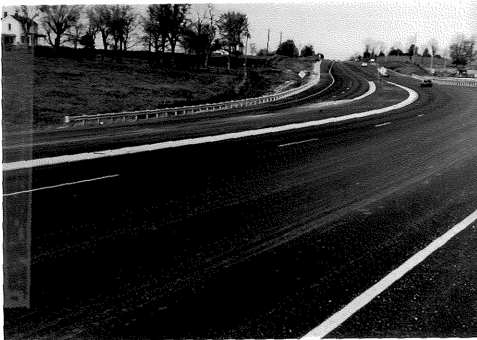
Figure 2. Overall View of Northern End of Project.
