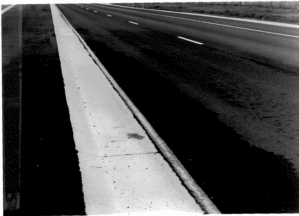
Figure 4. Overall View of Raised Median, Southern End.
