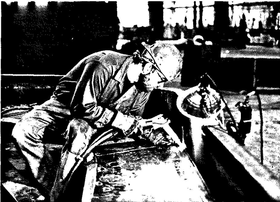
Figure 9. Manual SAW Used in a Short Weld Repair (Note Transducer Assembly on Backside of the Flange on the Right Corner of the Photograph).
