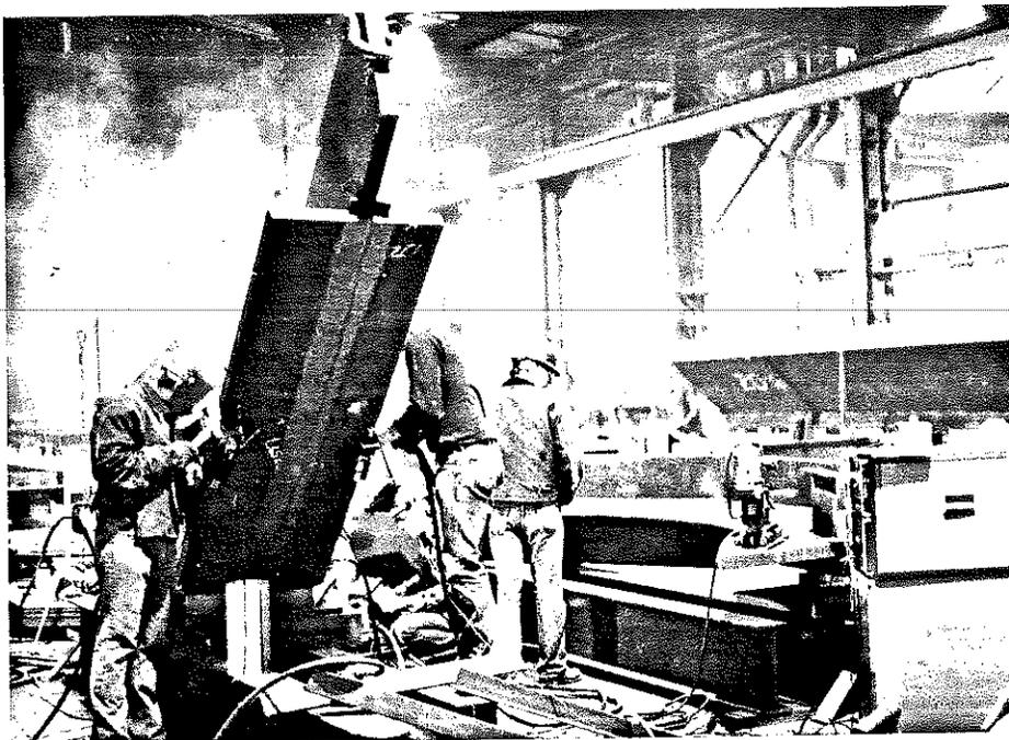
Figure 10. Concurrent Stiffener-to-Flange Welding with Transducers Located Opposite the Welds on the Backside of the Flange (Note the AEWL Located in the Right Corner of the Photograph).
