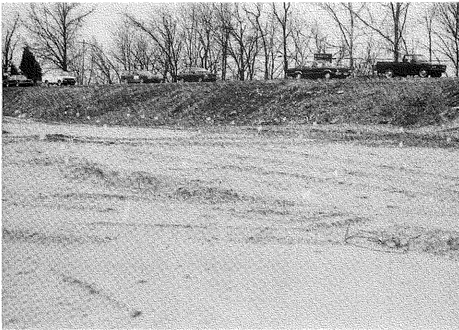
Figure 10. Flagged Wick Drain Layout.
