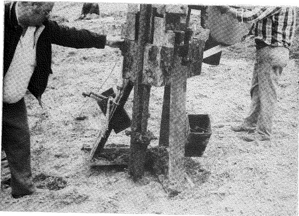
Figure 7. Wick Drain Being Located at Flagged Spot.
