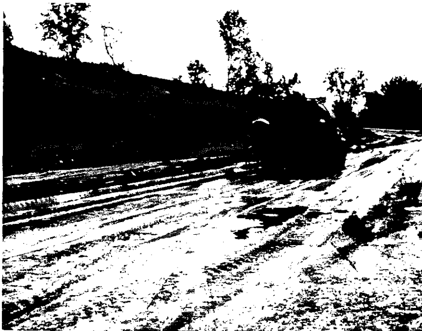
Figure 2. Applying the Curing Seal
