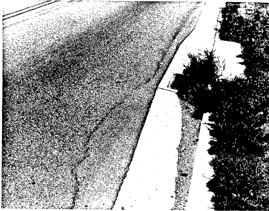
Figure 4. Shrinkage Cracking around Concrete Inlet Drain
