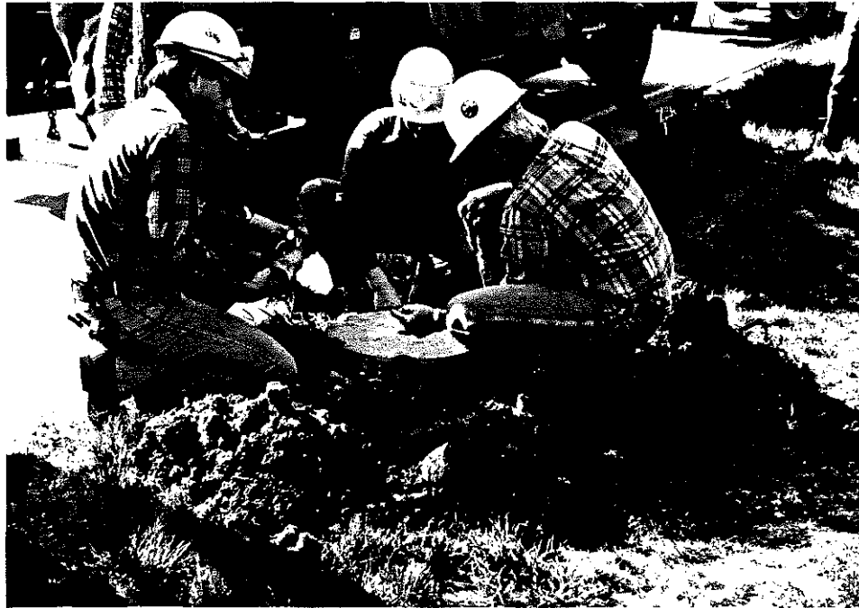
Figure 10 - Install Lower Tube with Base
