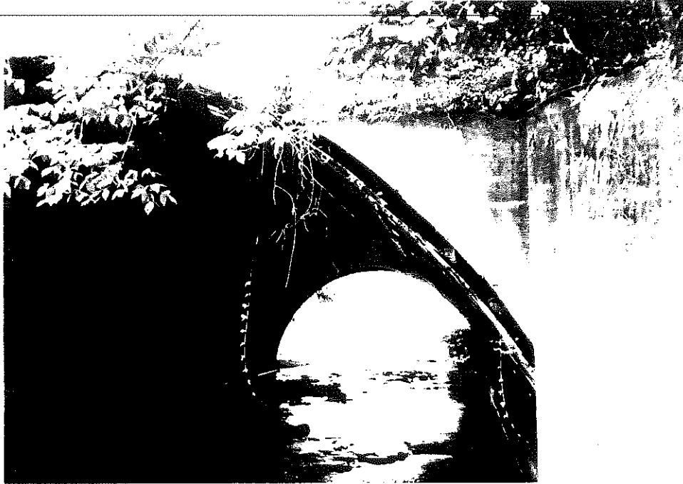
Figure 16. Lateral Displacement Observed between Headwall and Culvert Wall.
