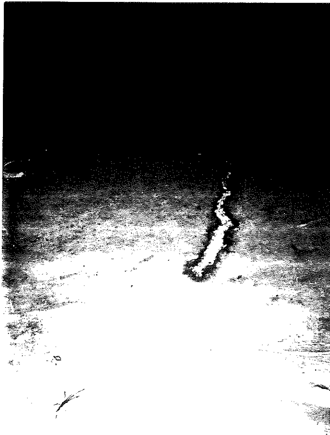
Figure 3. Cracking in Top Slab of Precast Box Culvert on KY 1934, Milepost 0.5.
