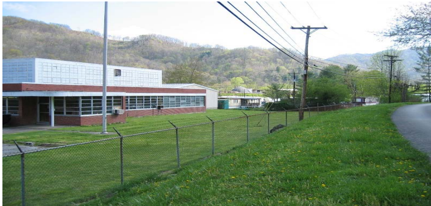
Figure 1.1. Site of NEC/Cooper Industries (now National Electric Service Company); Holiday Mobile Home Park can be seen immediately beyond the building and separated by a chain link fence.
