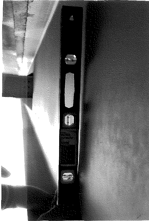
Figure 4. Measurement of Transverse Tilt on a Beam.
