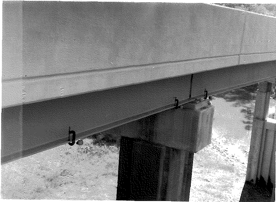
Figure 2. Optical Targets on Lower Flange of a Beam.
