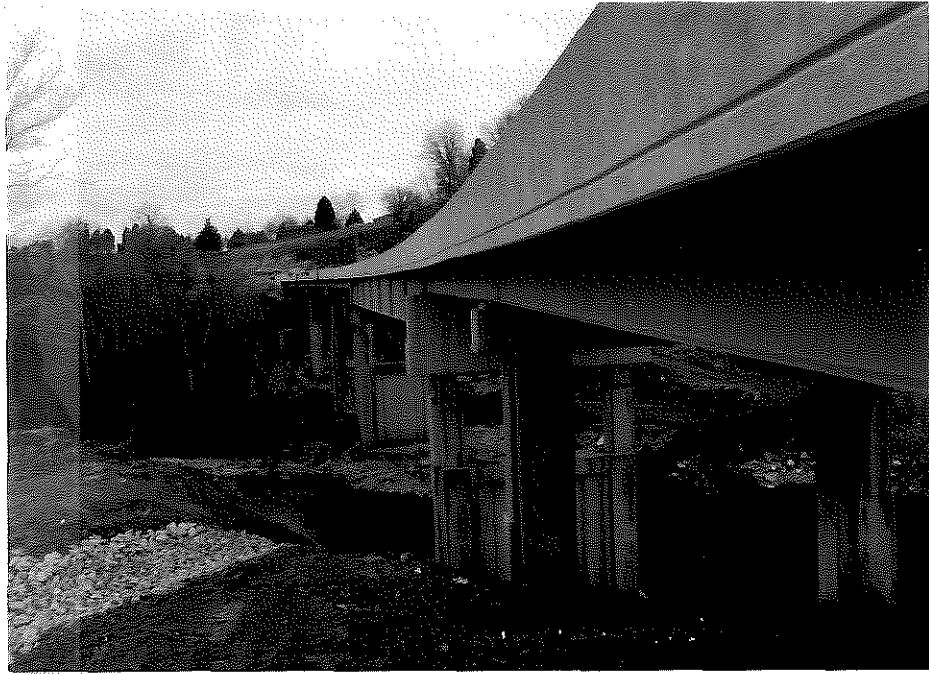
Figure 1. Six-Span Composite Steel Beam Bridge on KY 52 at the Boyle-Garrard County Line (Facing Westward).
