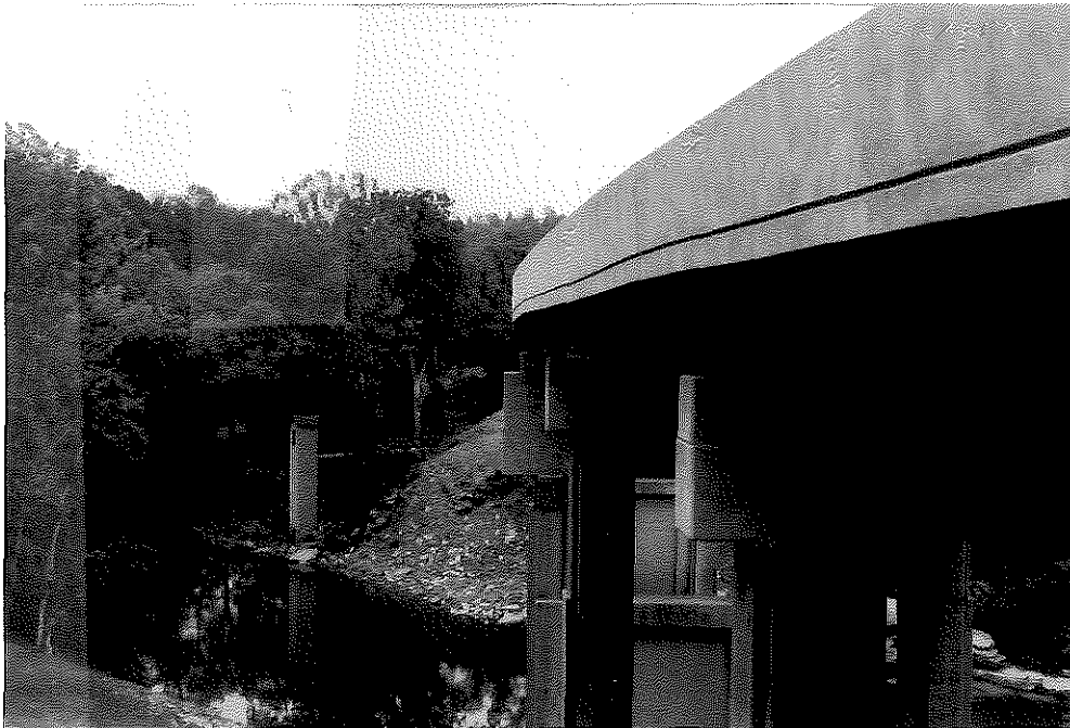
Figure 5. Rustication Groove in Spans 5 & 6 (Facing Eastward).
