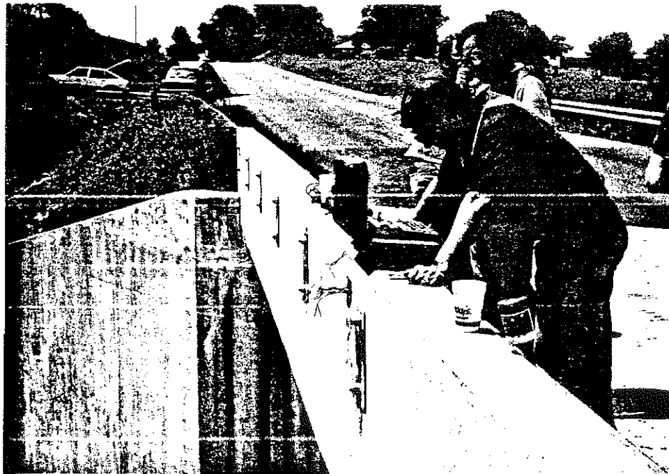
Figure 8. Polarization Resistance Measurements Being Taken of the Reference Electrodes Buried in the Deck of the Gose Road Bridge (July 24, 1987).
