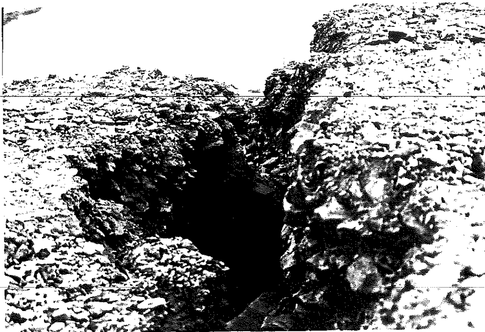
Figure 9. Failed Wall with Tension Cracks.
