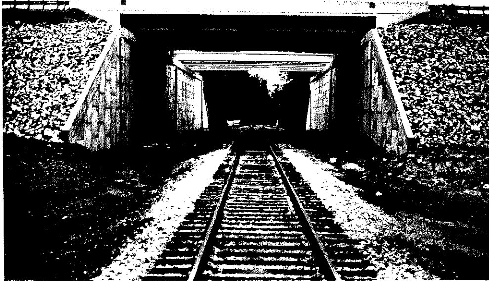
Figure 7 . Completed Structure with Southbound Lanes in Foreground.
