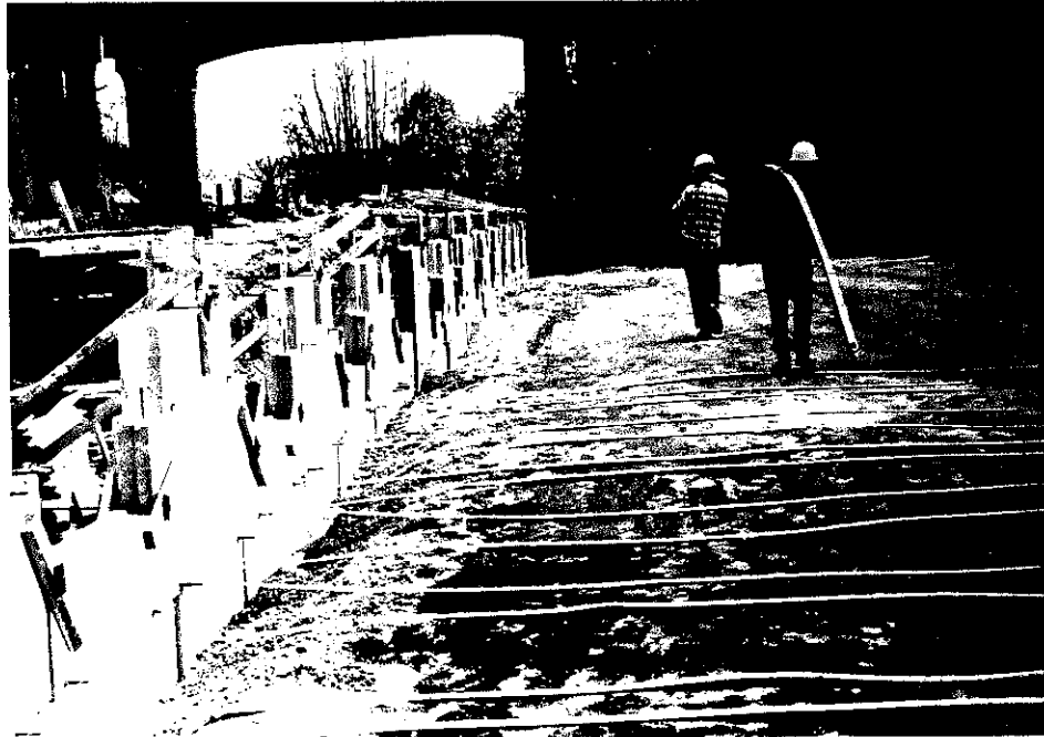
Figure 6. Construction of Reinforced Earth Wall with Supporting Straps in Granular Backfill.
