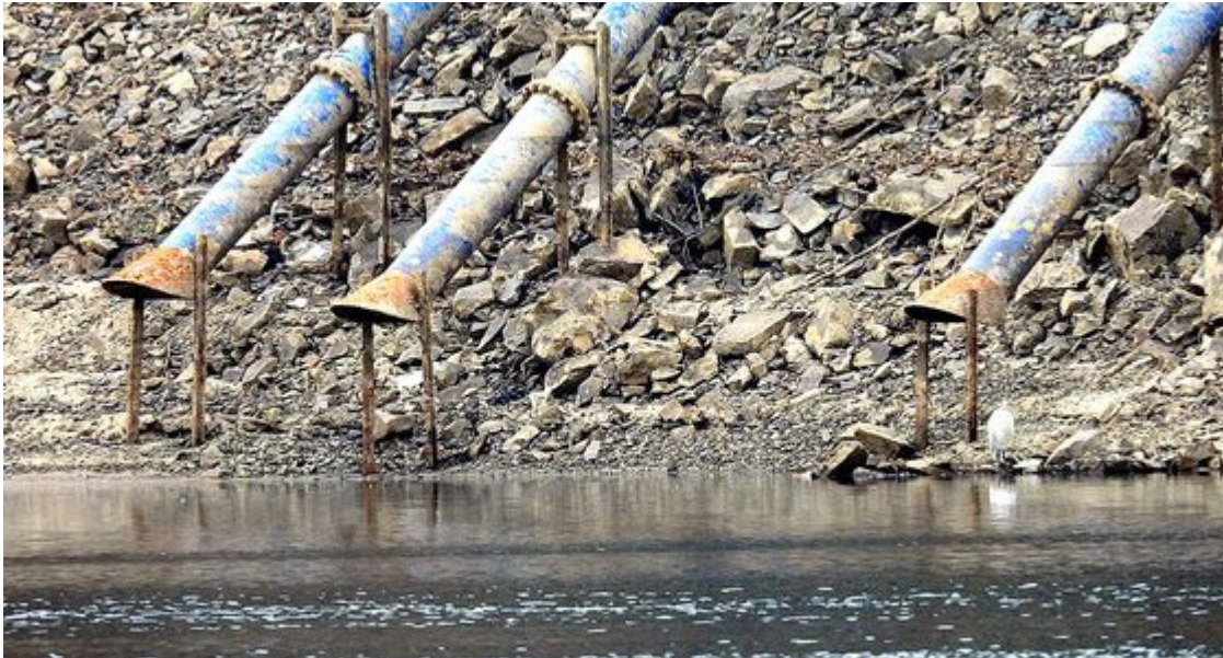
Figure 16 An example of a pumping constraint water level. The opening of the Hapcheon Changnyeong Weir on the Nakdong River in January 2022 reveals the intake of an agricultural pumping station upstream. (강찬수, 2023)
