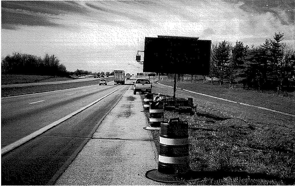
Figure 1. Variable Message Sign Equipped with Radar Unit.
