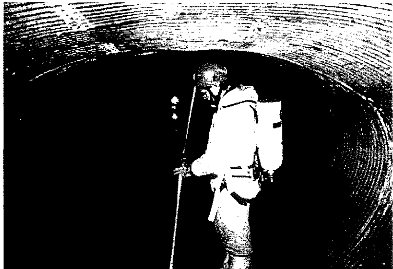
Photo 12. Joint 25, up grade
