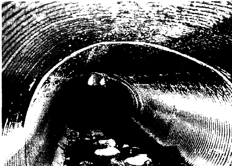
Photo 3. Joint 3-Joint 4, Pipe protruding into crown.
