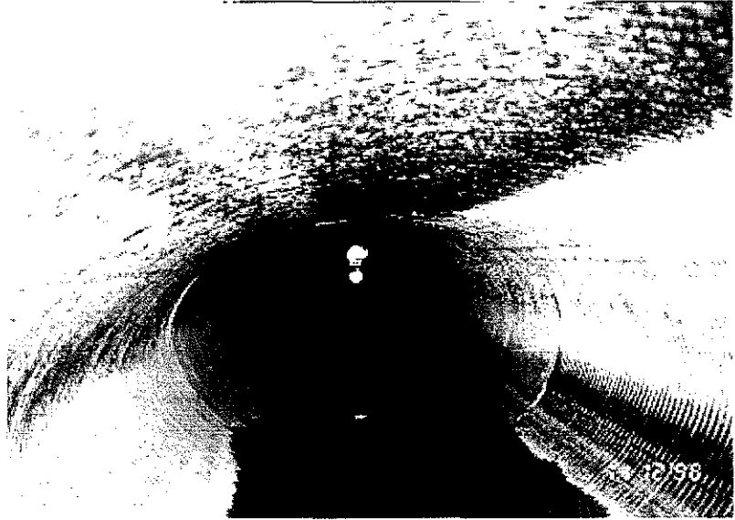
Photo 9, Joint 16. Pipe Elliptical
