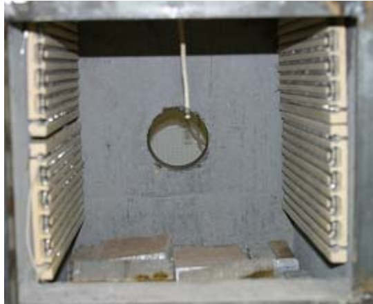
Figure 5.11 Furnace Interior- Electric Heaters, Scrap and Exhaust
