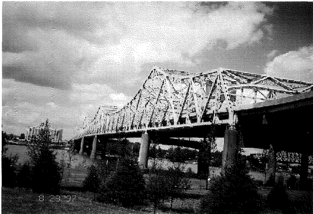
Figure 4. The I-65 (Kennedy Bridge) bridge over the Ohio River.
