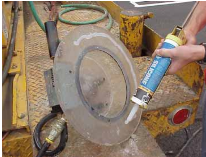
Figure 8. Placement of Silicone Bead.
