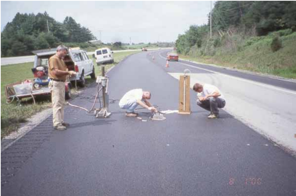
Figure 13. AIP Reading and Coring at Test Site.
