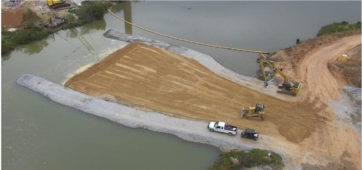
Figure 3. Aerial view of divider berm construction, north is on the left.
