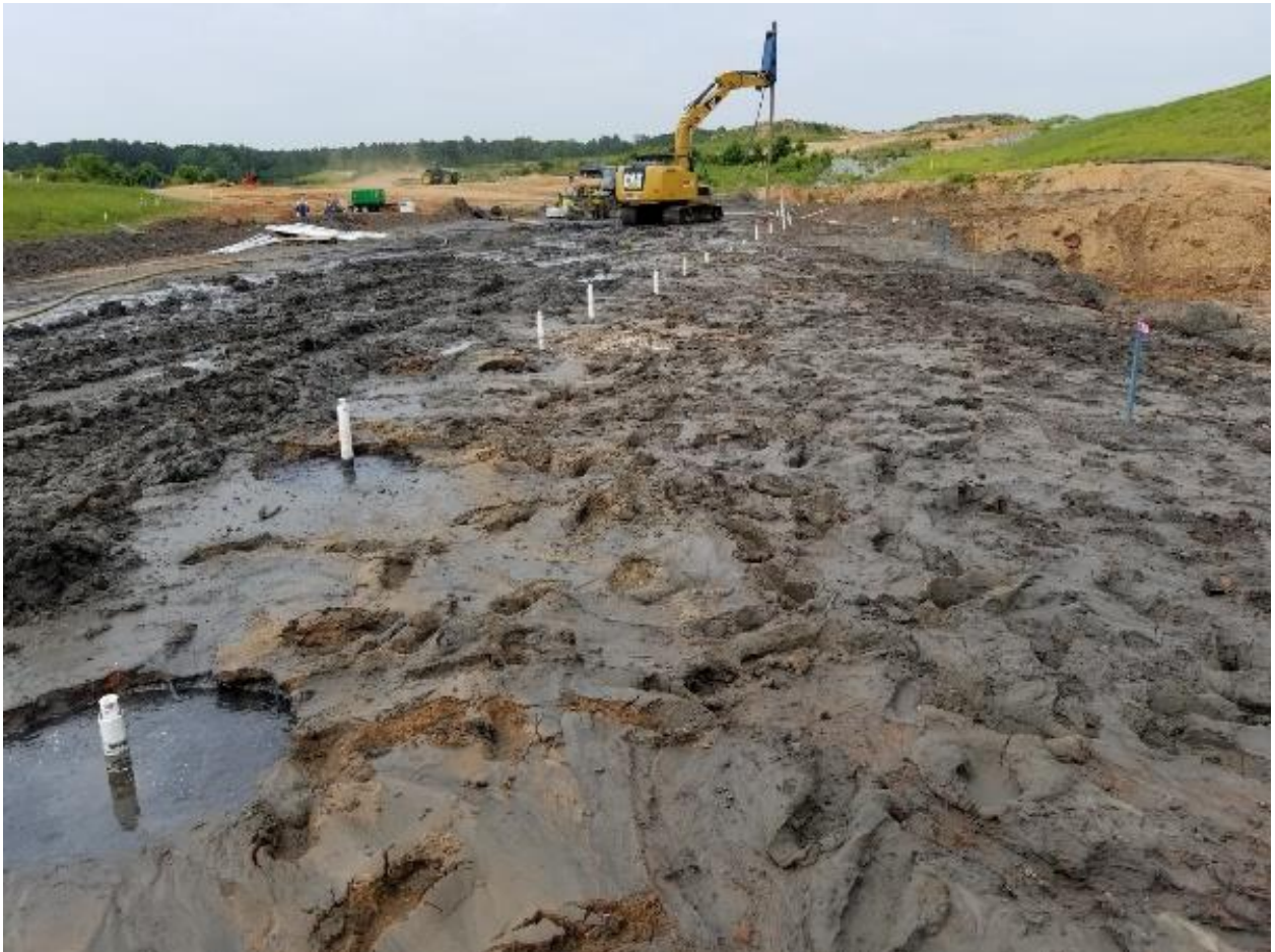
Figure 10. Site conditions prior to dewatering.
