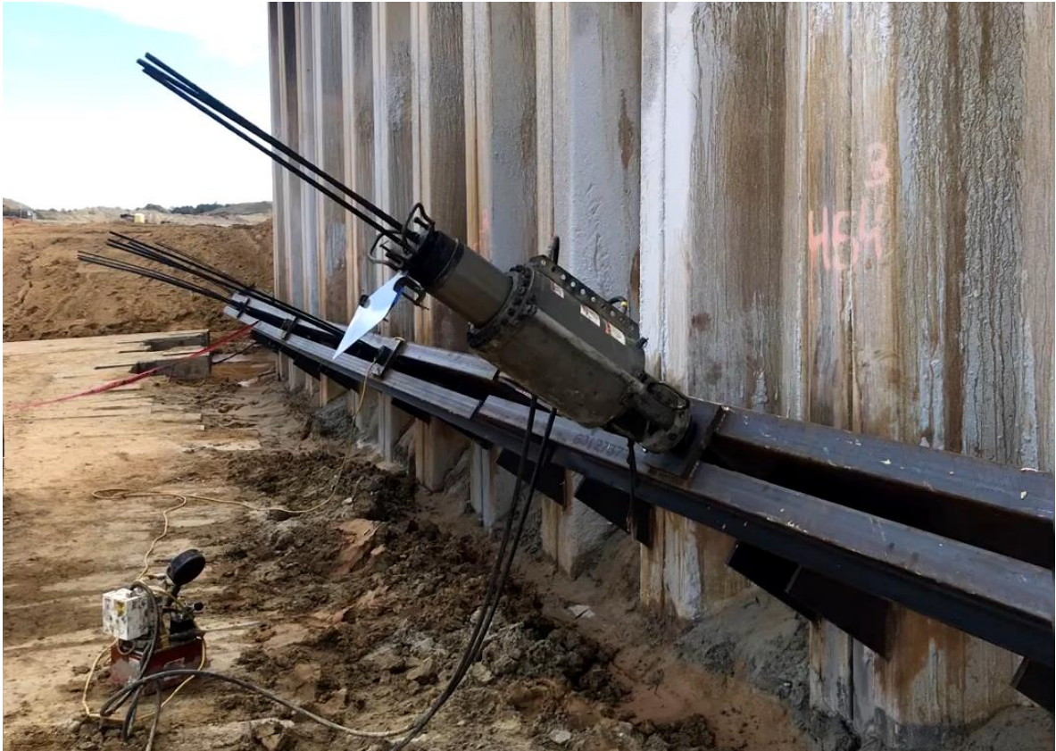
Figure 8. Anchor testing and lock off in process.
