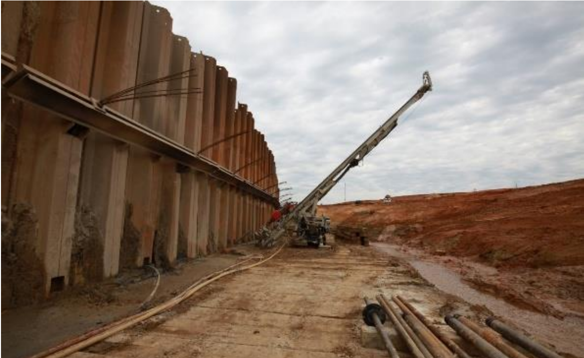
Figure 7. Drilling the second row of anchors.
