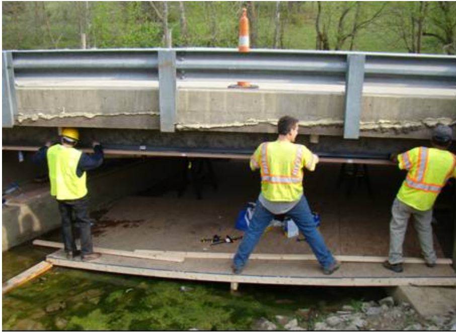
Fig. 5.20: Placing laminate on the top flange
