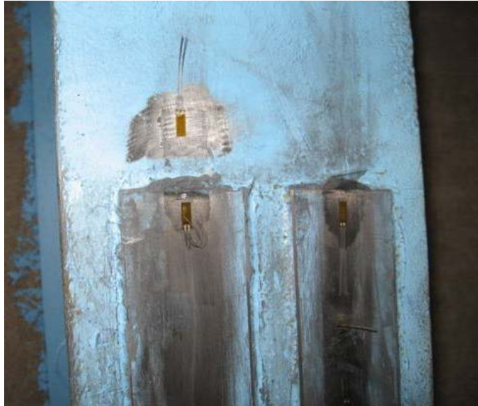
Fig. 5.29: Attached strain gages on the two bottom laminates on girder G3
