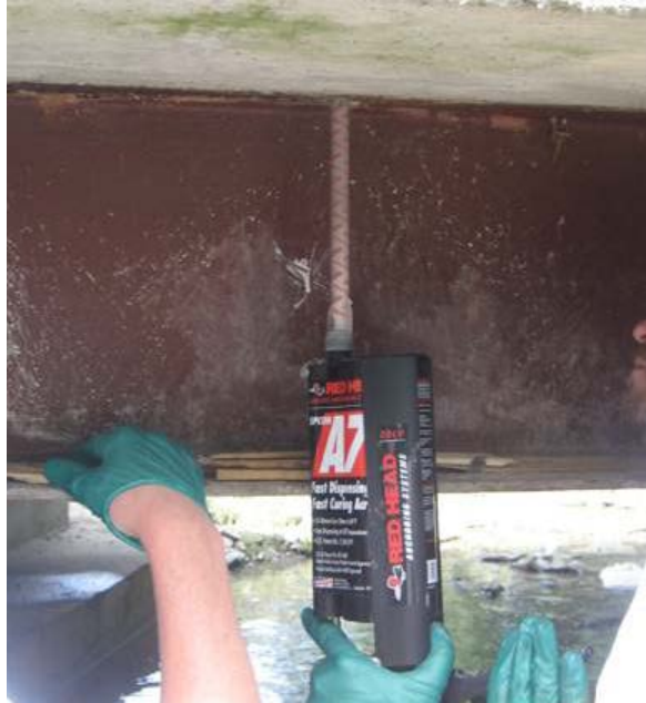
Fig. 5.9: Inserting of adhesive into drilled hole
