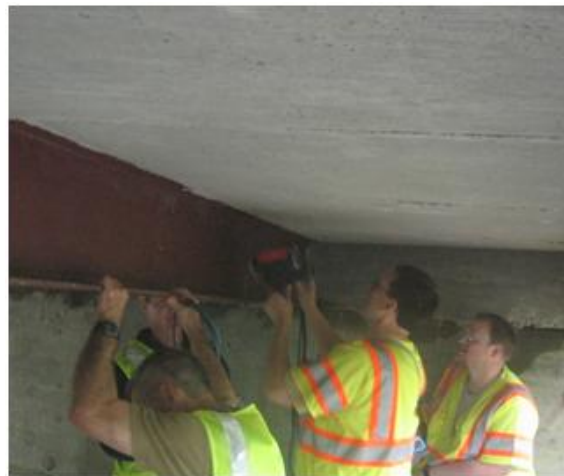
(b) Locating rebar positions on the bottom surface
