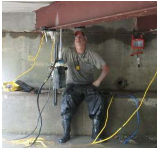
Fig. 5.7: Drilling rig fixed to the bottom flange
