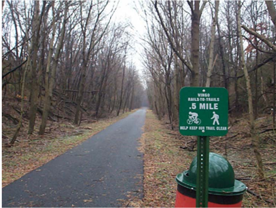
Figure 2.3: Wingo Rail Trail near Mayfield in western Kentucky
