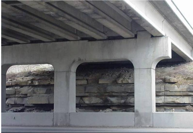
**Figure 3.** Example of AASHTO-Type Prestressed Concrete I-Girder.
