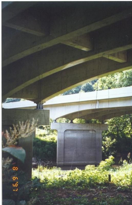
**Figure 4.** Example of Concrete Intermediate Diaphragms in Bridge with Haunched Girder.
