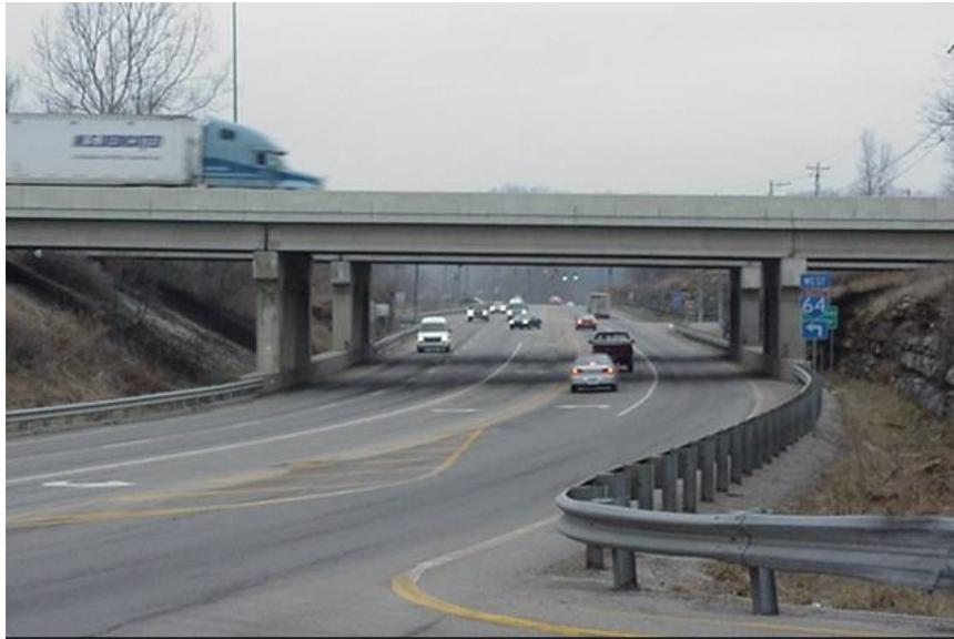
**Figure 12.** Prestressed Concrete I-Girder Construction of I-64 Bridge over KY32.
