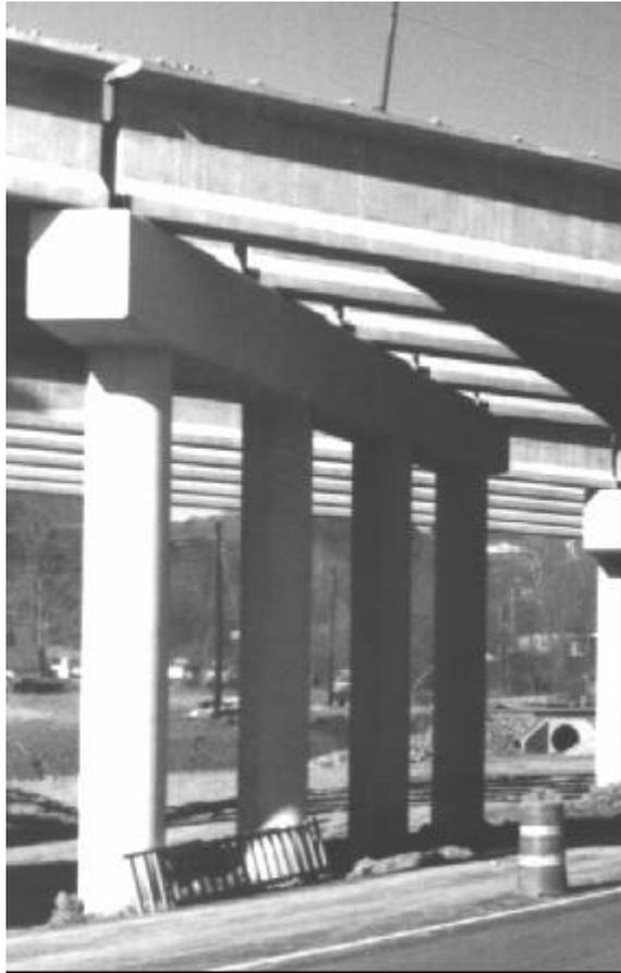
**Figure 5.** Skew of Bridge Girders Relative to Pier Support.
