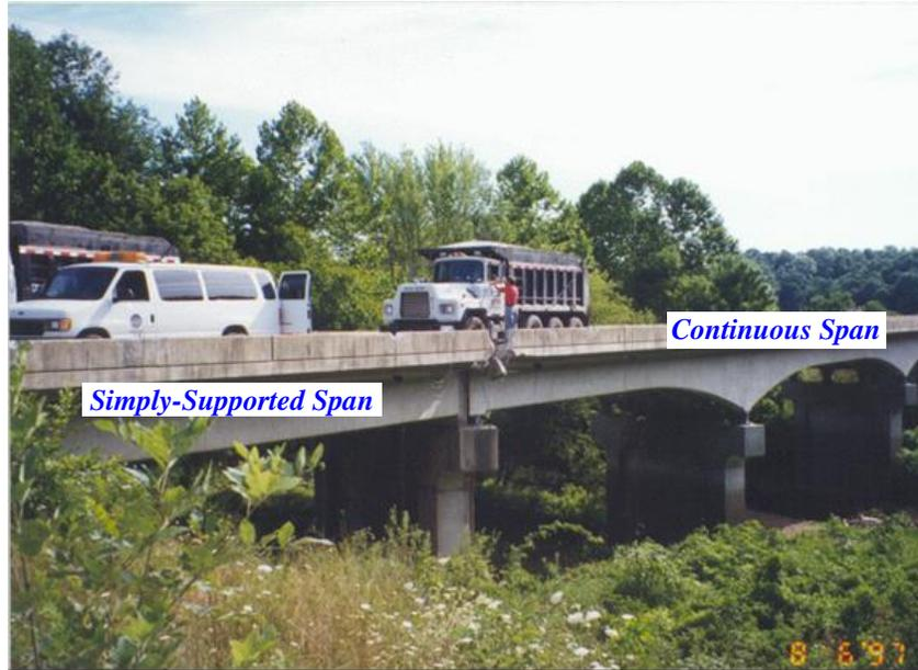
**Figure 31.** Haunched Girder Construction of I-64 Bridge Over Triplett Creek.
