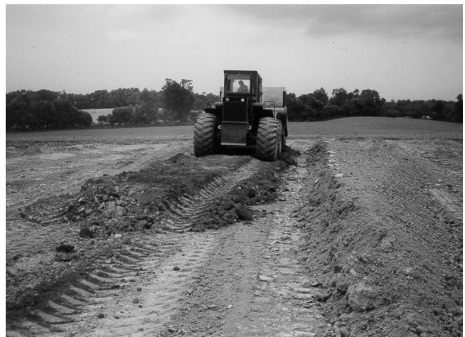
Figure 7. Scraper constructing a windrow of soil.
