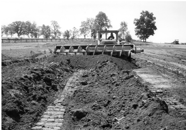
Figure 8. Front view of soil regenerator making second pass.
