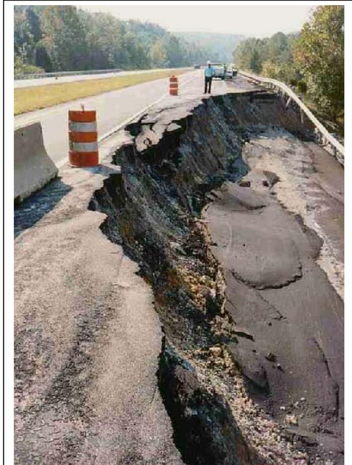
Figure 1. Massive highway embankment failure on a parkway route in Butler County—repair cost was 1.4 million dollars
