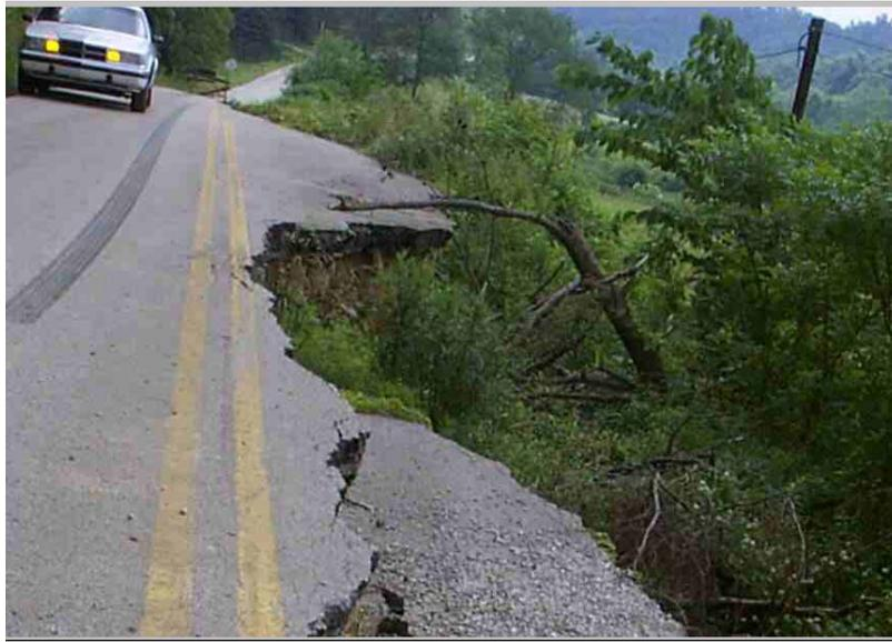
Figure 6. Highway embankment failure on KY 847 in Owsley County
