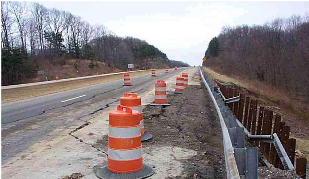
Figure 7. Attempts to halt highway failure using railroad steel rails
