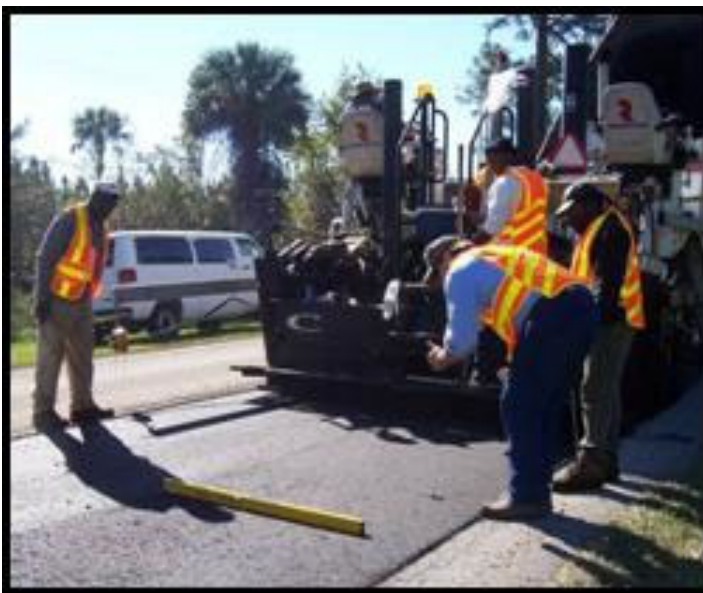
Figure 1.2 Inspection of Asphalt Material (From FHWA, 2020c)
