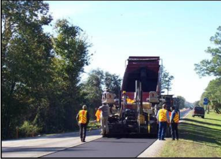
Figure 1.1 Contractor Paving Crew placing Asphalt Material (From FHWA, 2020c)
