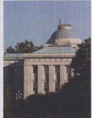
NC Capital Building
