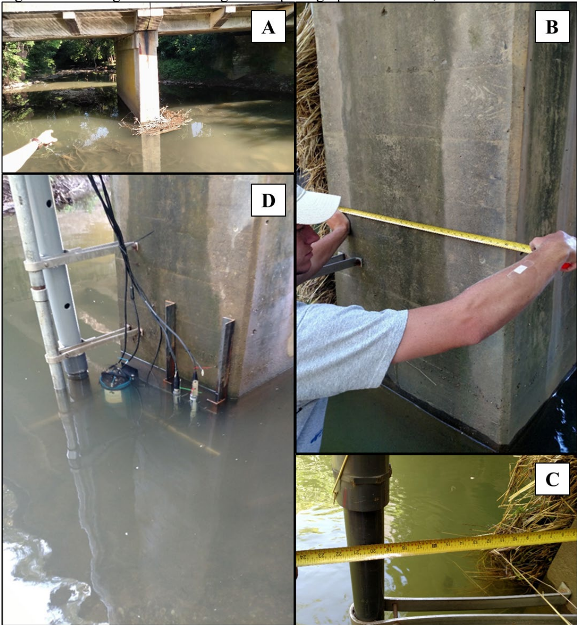
Figure 4.3 SE Gage sensor site. Figure and photographs from Clare, 2019.
