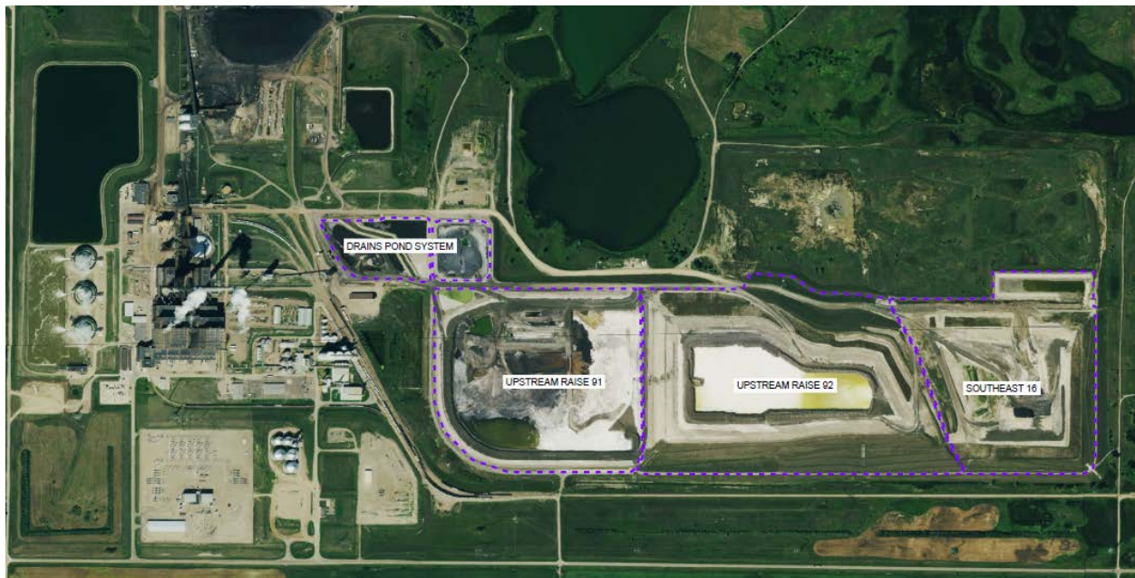
Figure 1. Coal Creek Station and Upstream Raise 91 CCR Surface Impoundment.
