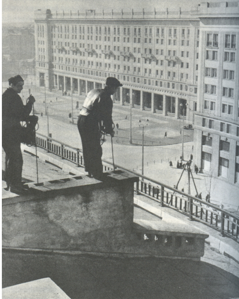
Figure 3.3. Marszałkowska Housing District (Marszałkowska Dzielnica Mieszkalna) and Constitution Square. From Crowley, David. Warsaw , Topographics. London: Reaktion, 2003, 116.
