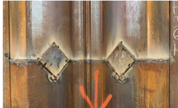
Figure 5. Face View of a Completed Splice on a Sheetpile Pair.
