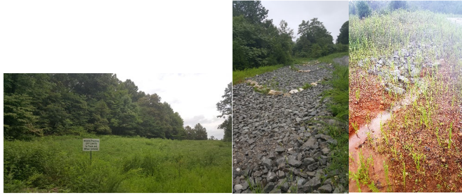
Figure 1.2 Fort Knox restoration efforts, images taken by Cara Peterman. Images from left to right: Fort Knox Training area, restoration using native grasses. Fort Knox erosion control method, using riprap to slow soil erosion and transport, newly installed. Fort Knox older erosion control riprap with some erosion present. Fort Knox, Kentucky.
