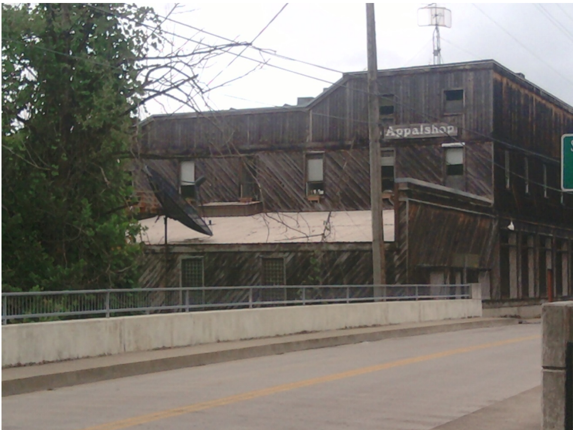
Figure 21 Appalshop headquarters from the Boone Building across the bridge over the North Fork of the Kentucky River, Whitesburg, Kentucky, July 9, 2014 (photo by author)
