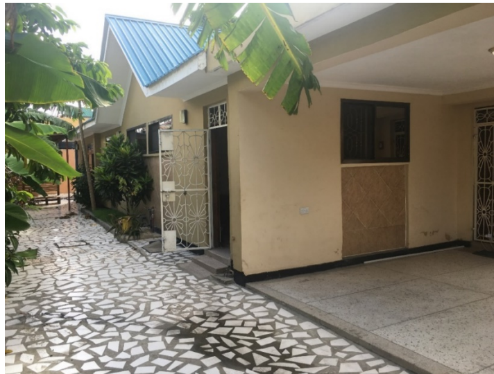
Figure 4. Outside of Tai Tanzania main office building
