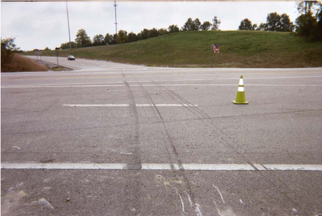
Skid marks on pavement caused by semi.
