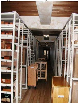
For better air circulation and a drier environment, the south and north sides of the basement are exposed to outside air.
