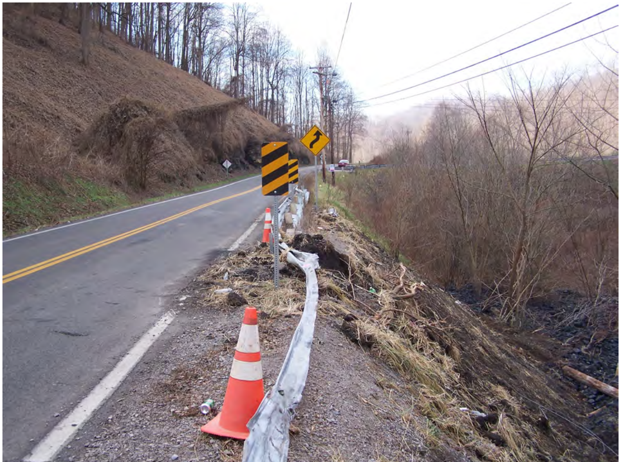
Location where tractor and trailer came to rest. Photograph taken by KY FACE personnel.
