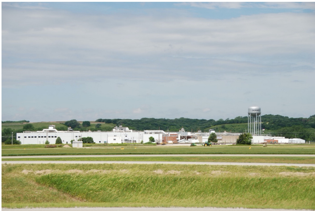
Figure 7. From transect across Northwest Iowa: Stage 3–Treading Water. Meat processing plant in Cherokee.
