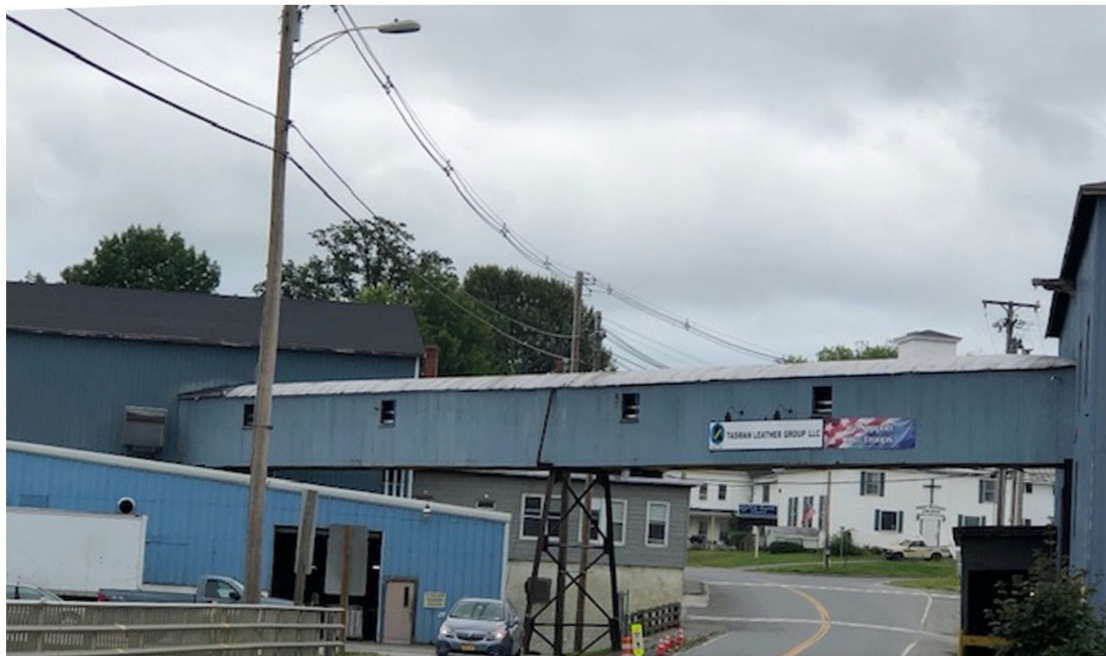
Figure 12. From transect across Central Maine: Stage 3—Treating Water. Route 43 passing through the Tasman tannery complex in Hartland, Maine. (Photo courtesy of Betty Austin).
