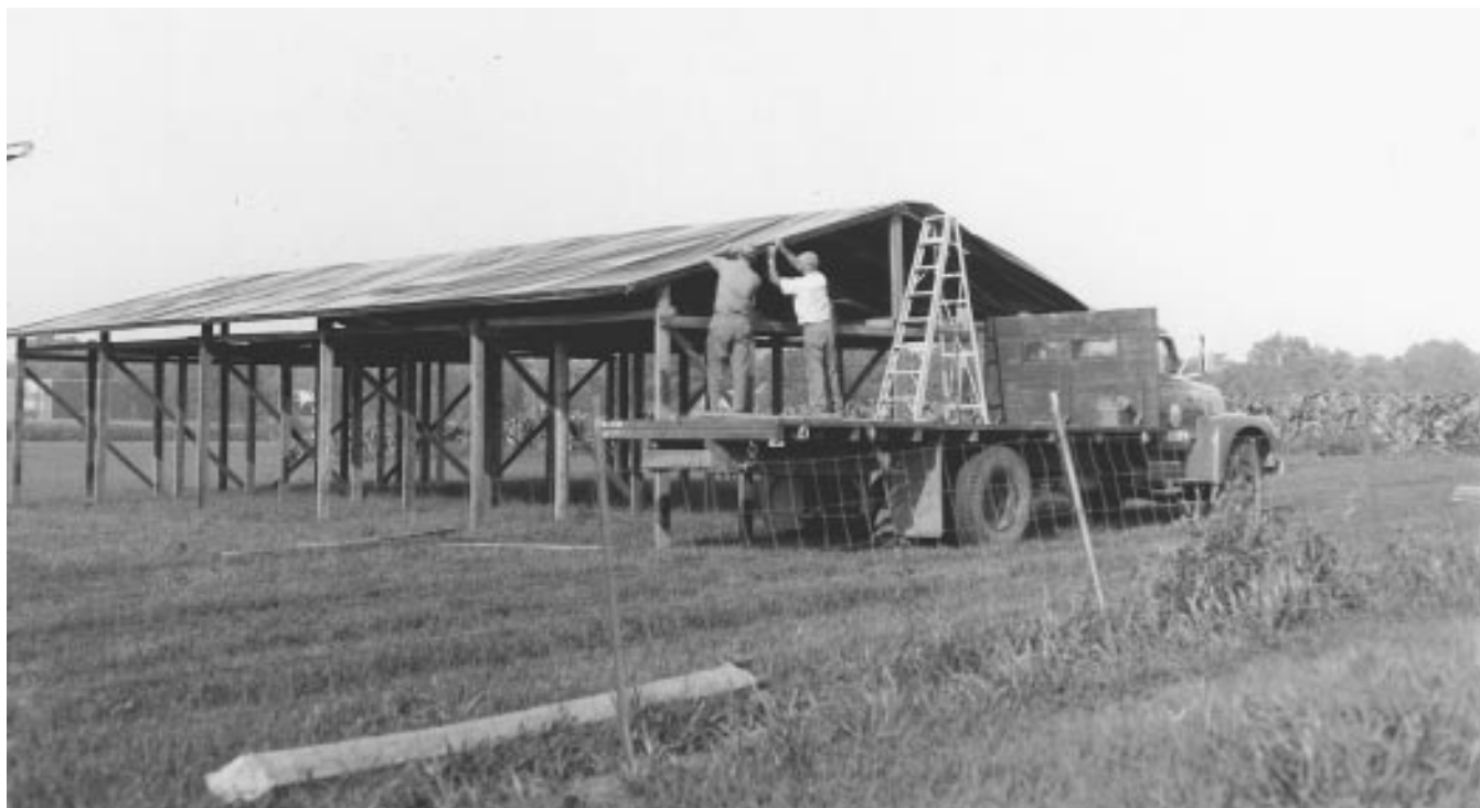
Figure 1. Construction of a pole-type plastic-covered curing structure.
