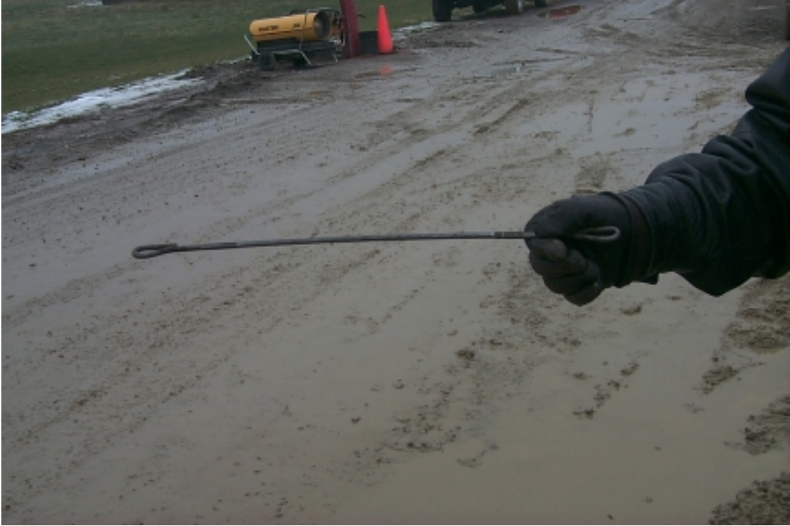
Picture of wire used for horizontal stability of concrete form.
