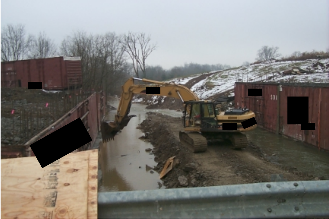
Picture of track hoe used to pull concrete away from worker.
