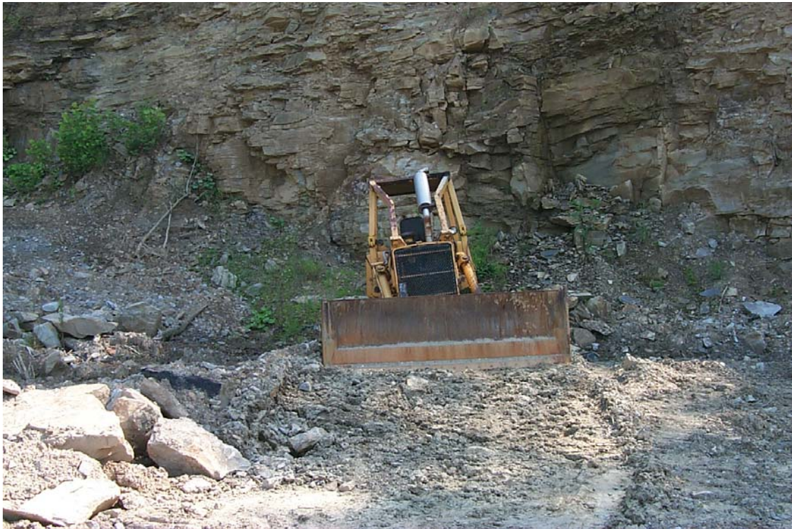
Bulldozer in the side of the mountain.
