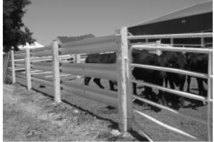
Figure 15. Holding pen with sidewall made from guardrail.
