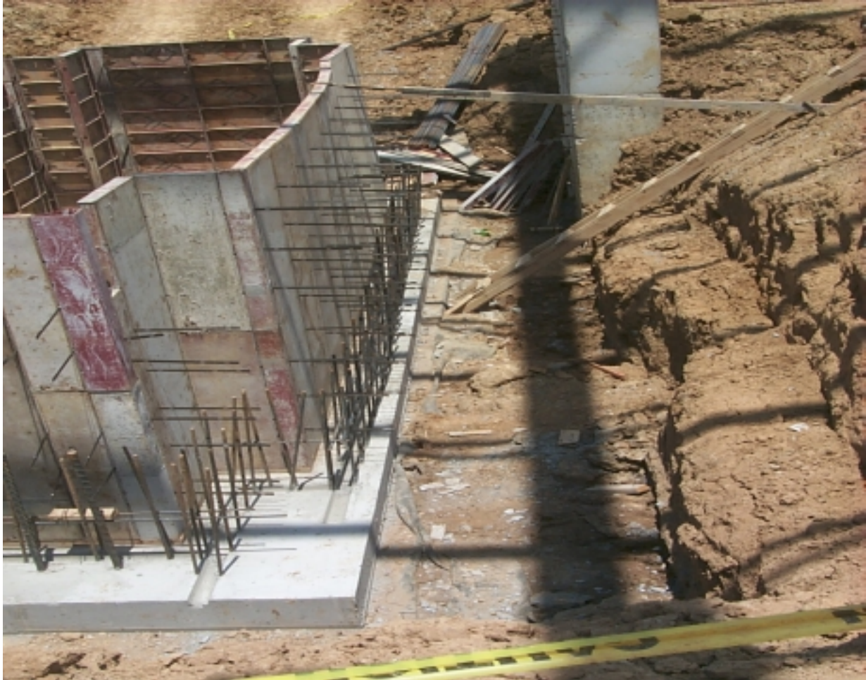
Victim helped make wooden forms for concrete pad.
