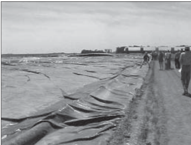
Figure 3. Anchor trench on impermeable plastic installation.
