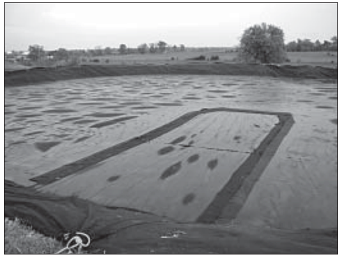
Figure 6. Opening for the access of agitation and pumping equipment in a geotextile-covered manure storage.
