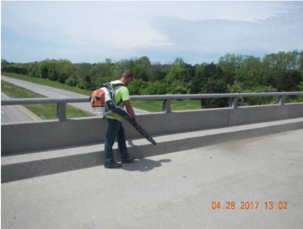
Figure 3 Removing debris with leaf blower
