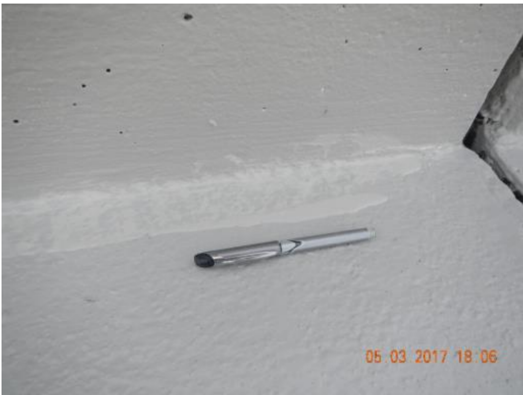
Figure 8 Excessive runs
