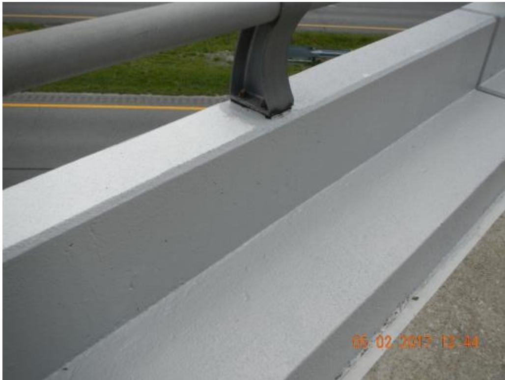
Figure 7 Top of barrier wall with no top coat
