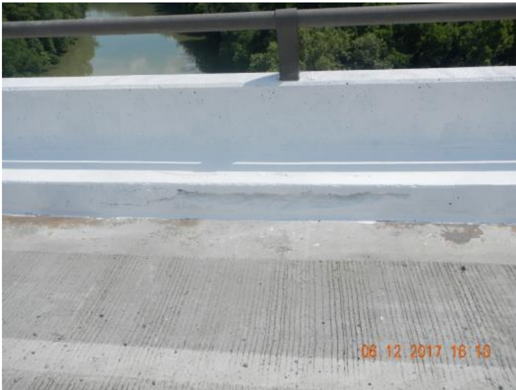
Figure 12 Spalled concrete
