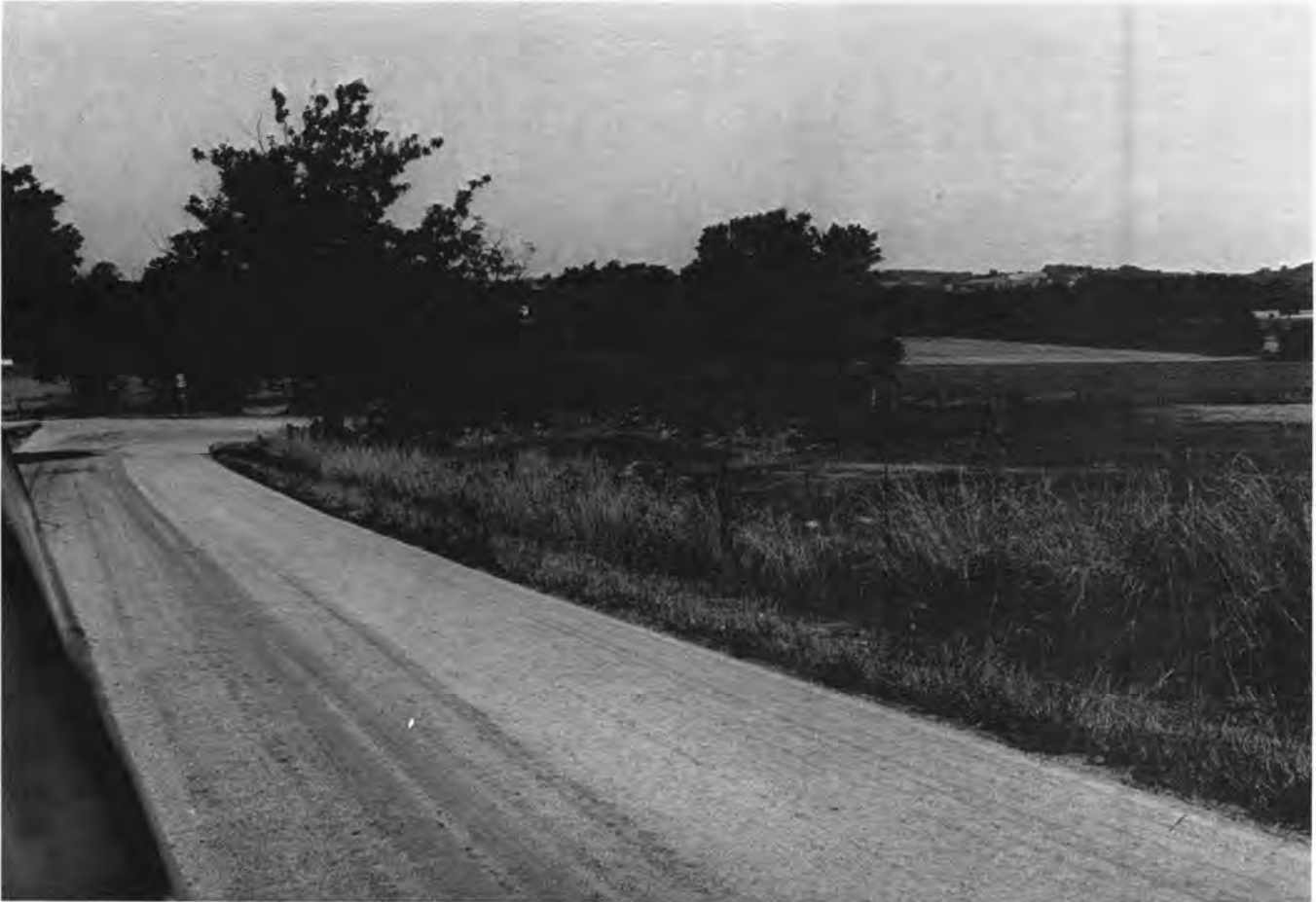
Figure 11. Agricultural development obscures the Shropshire Vein, Woodford County.
