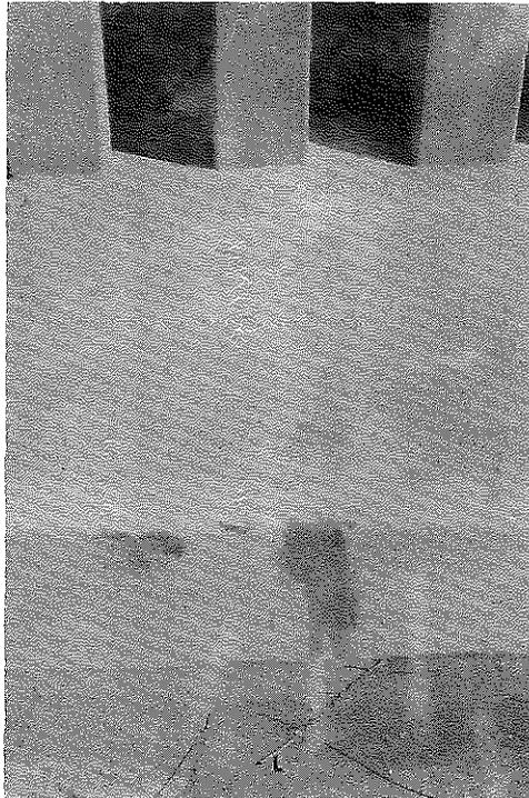
Fig. 8. This is a Typical Crack After the Resin and Sand has been Applied and the Mixture Flattened out to Fit the Contour of the Existing Concrete.
