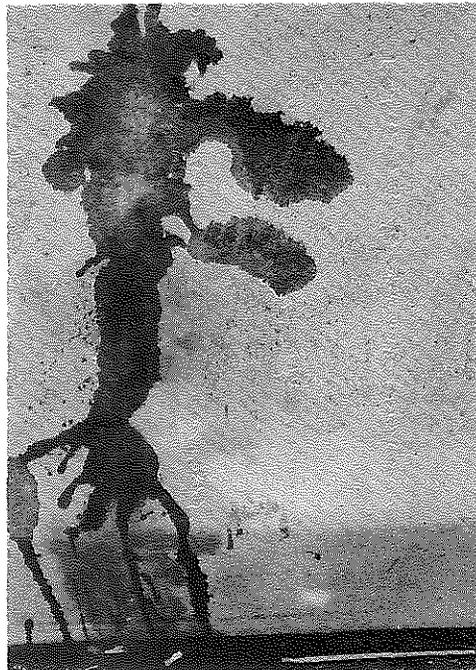
Fig. 17. This Close-up of a Flooded Crack Showed the Effect Obtained with a Thicker Coating of epoxy and sand. The crack was well sealed as evidenced by its refusal to allow ingress of water.
