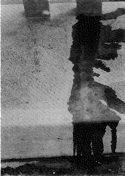
Fig. 16. This is a Typical Crack After 6 Months Service which was Flooded to Detect any Seepage. No water entered the crack and its water tightness was verified. The outline of the crack can be seen here through the thin covering of transparent resin. If it had been possible to apply more sand before the swath of resin hardened the sealed crack would not have been visible. However, the crack was sealed and the concrete and steel protected.
